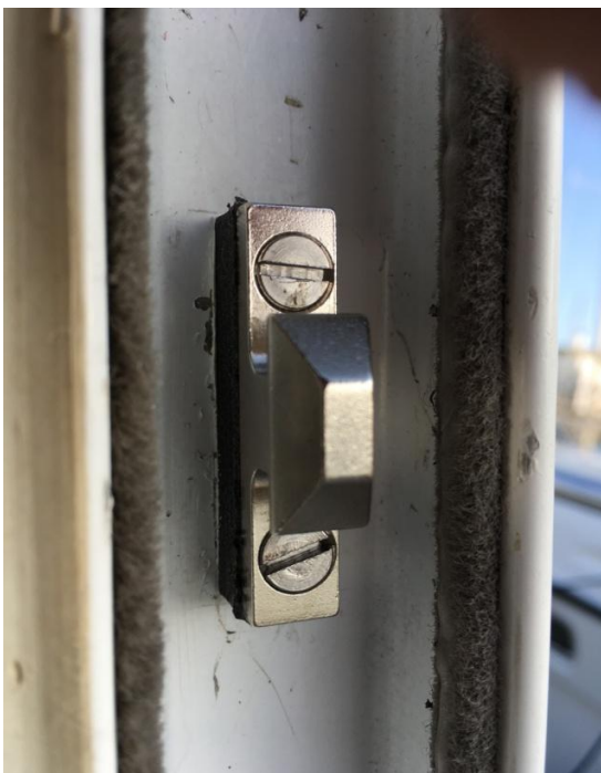
inside when finished
