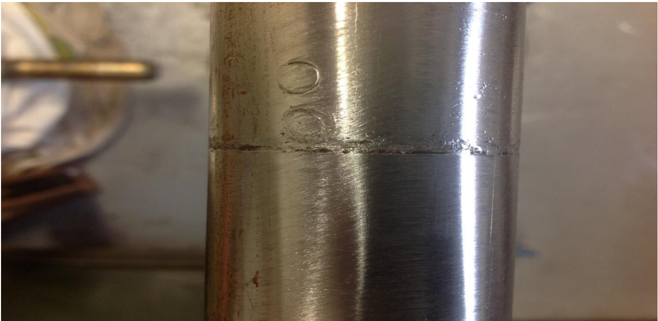
This shows the port shaft damage: a ring of corrosion and dimples from the grub screws of a previous seal type. No lip seal could hope to seal against this damage.
